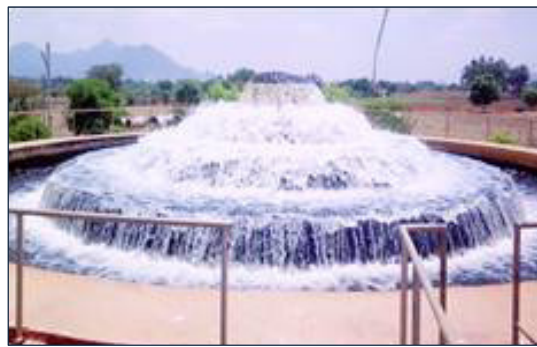
b) View of the Cascade Aerator
